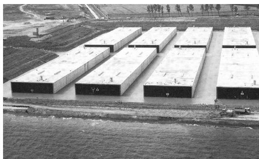
Pic. 2. Tunnel elements in dry dock.
