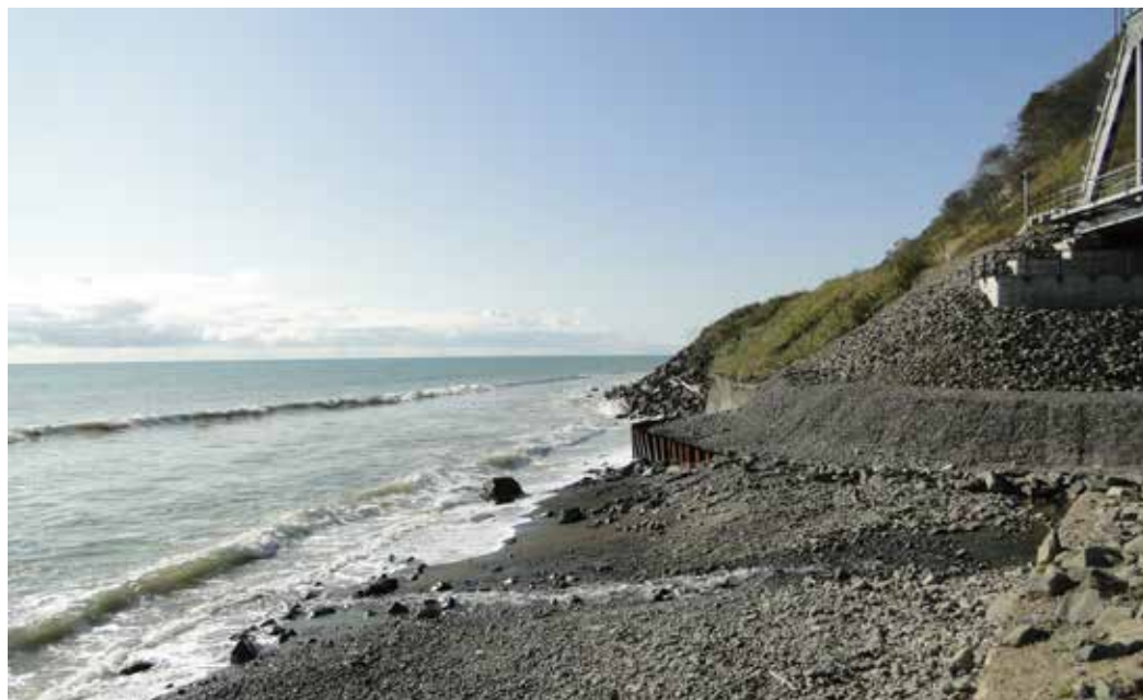
Pic. 1. Washing away of the bridge abutments at 263 rd km of Korsakov – Nogliki section of the Far Eastern Railway. 2020 [photo made by the authors].
