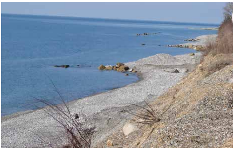
Pic. 3. View of deformed stone spur dikes [photo by the author, 07.02.2008].
