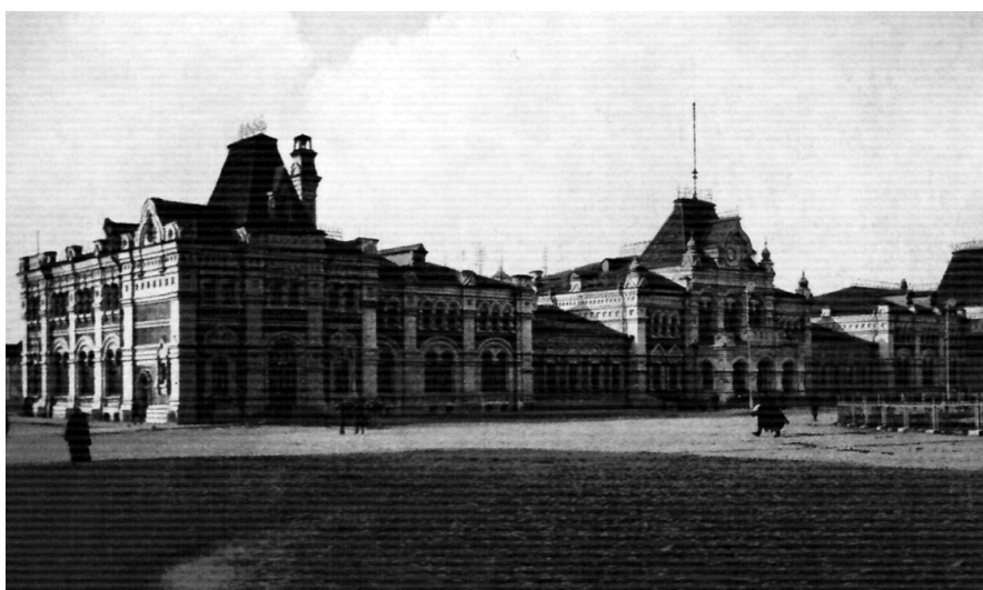
Pic. 20. Vindavsky (now Rihzsky) railway station.
