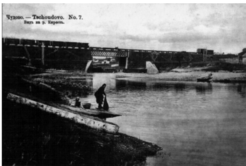
Pic. 14. Railway bridge at Chudovo station.
