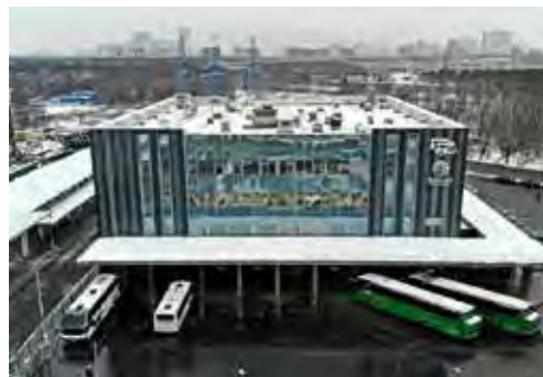
Pic. 7. Khovrino Transport Interchange Hub. Severnye Vorota bus station.
