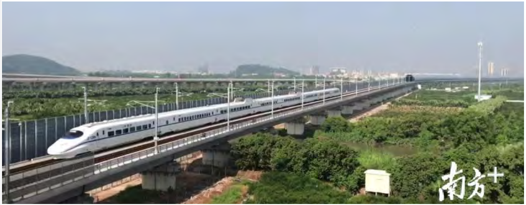
Pic. 1. HSR overpass of low height in China ( http://news.southcn.com ).
