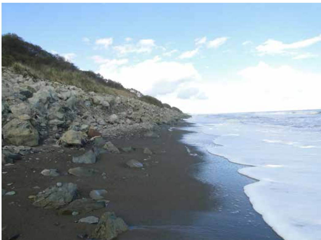
Pic. 3. Washing away of the base of the roadbed slope at 273 rd km of the section Korsakov – Nogliki. 2020 [photo made by the authors].
