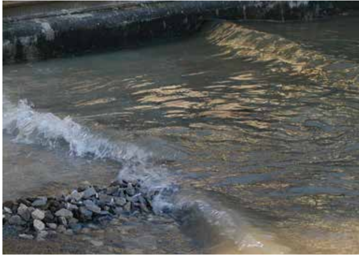
Pic. 5. Interaction of waves with the stone spur dike [photo by the author].
