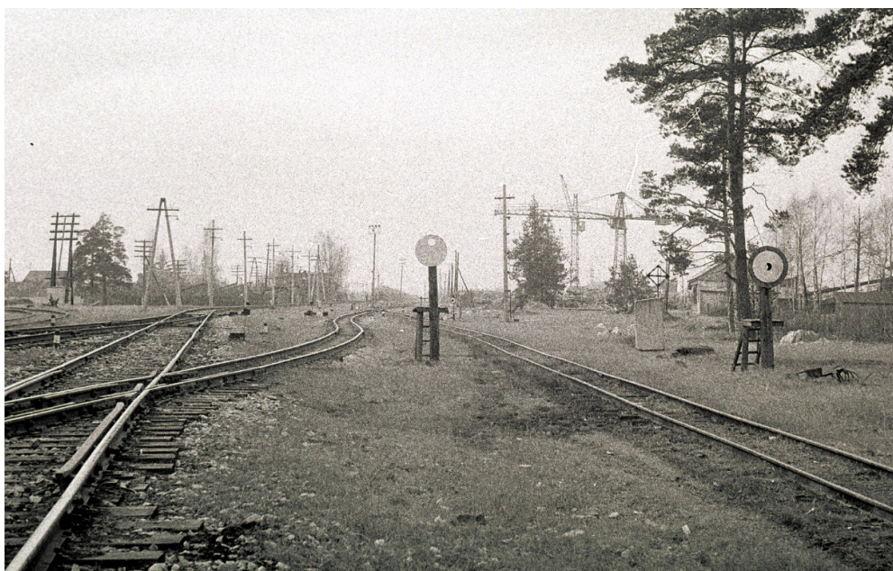
Pic. 13. Neck of Pilevo station. From right to left, there are hauls: Pilevo–Tyukovo, Pilevo–Spas-Klepiki narrow gauge line, Pilevo–Sorokovoy Bor normal gauge line. Photo by V. Mironov, published with his kind permission.
