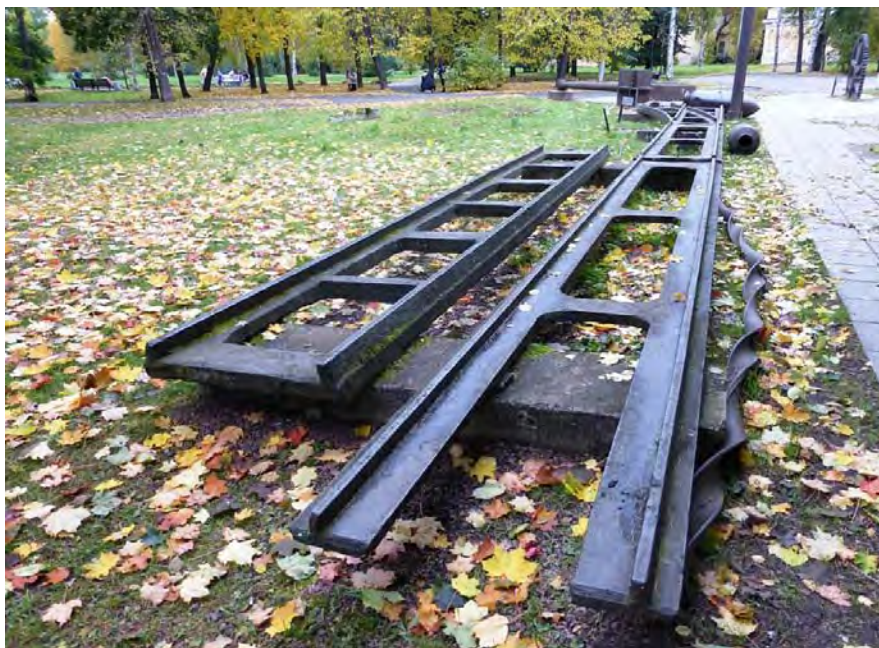
Pic. 1. Construction of the superstructure of the track "Cast iron wheel line". [Electronic resource]: https://umcздt.ru/news/demohtml/80.html . Last accessed 11.06.2021.
