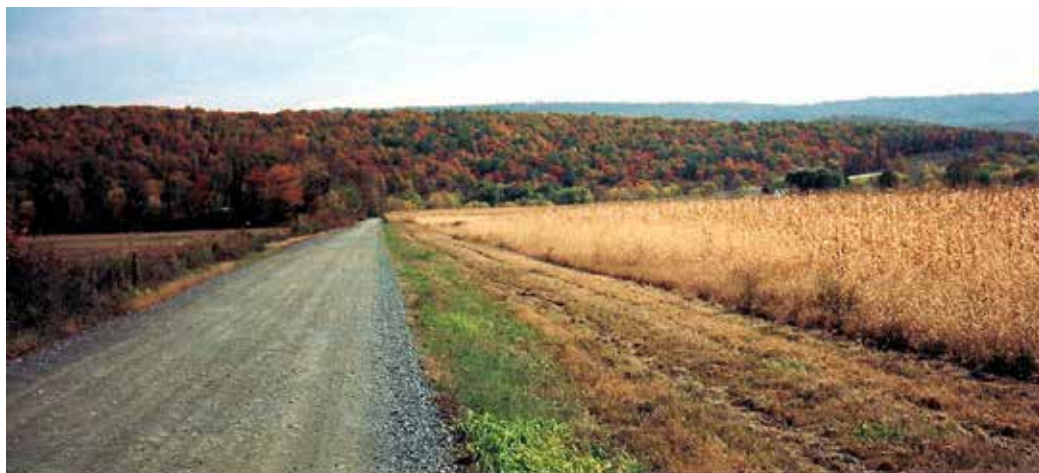
Pic. 6. Country road built using Macadam's technology (Macadam. [Electronic resource]: https://en.wikipedia.org/wiki/Macadam . Last accessed 11.06.2021).
