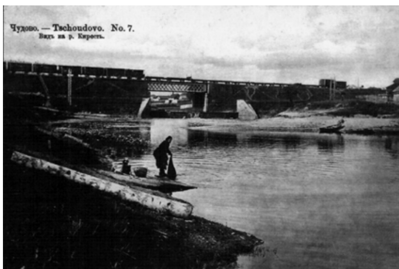
Pic. 14. Railway bridge at Chudovo station.
