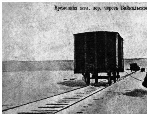
Pic. 7. Temporary railway laid on the ice of the lake Baikal.
