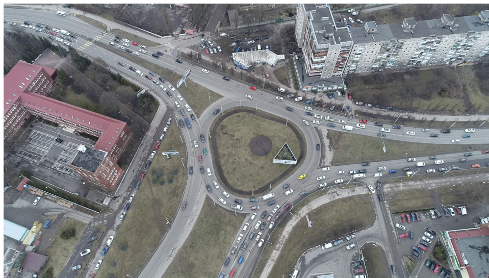
Pic. 1. Surveying a circular intersection from a quadcopter (provided by JSC Giprostroymost Institute).
