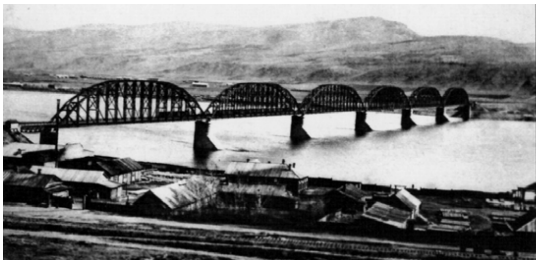
Pic. 11. The bridge across the Yenisei [6].
