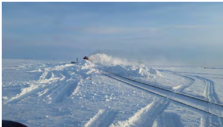
Pic. 12. Cutting of a snow hole using a FRES machine (photo by V. V. Shapran, 2015).
