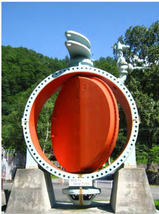
**Pic. 4.** A large shutter with a flat-blade disc used at a hydropower plant in Japan [1; 2]. [Electronic resource]: [https://commons.wikimedia.org/wiki/File:Yagisawa\\_power\\_station\\_inlet\\_valve.jpg?uselang=en](https://commons.wikimedia.org/wiki/File:Yagisawa_power_station_inlet_valve.jpg?uselang=en). Last accessed 22.07.2019.
