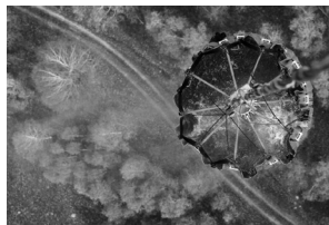
Pic. 1. Soft cylindrical tank with large rigid ring for water intake.
