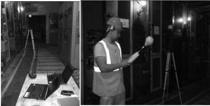
Pic. 1. Measurements of EMF at a traction substation.
