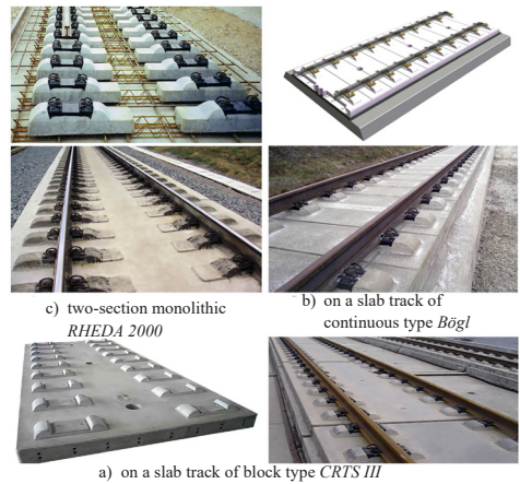
Pic. 1. Types of construction of a ballastless track superstructure.
