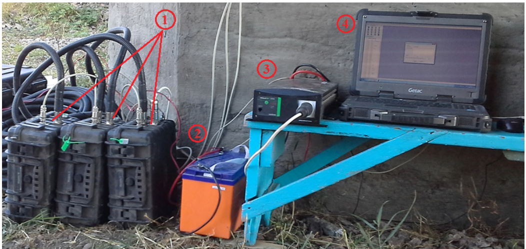
Pic. 3. General view of the mobile complex for tensometric measurements: 1 – measuring modules; 2 – rechargeable battery; 3 – sinusoidal inverter; 4 – a semi-industrial computer.
